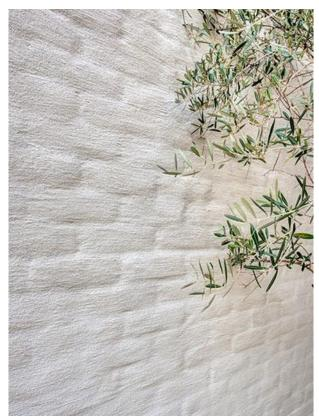
Example of KEIM Limewash mixed with Lime Slurry applied to a brick surface. Note that the slurry thickened Limewash fills in mortar joints and has a slight sandy texture.
